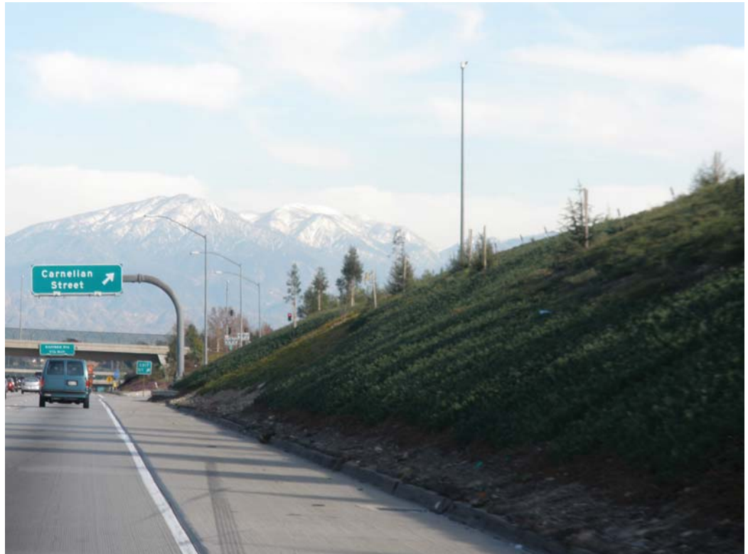
Berm along I-210 Freeway.
