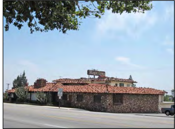
Fig 2: Magic Lamp, 8189 Foothill Boulevard (constructed 1941, elaborately remodeled 1956-57) (Chattel Architecture 2009)
