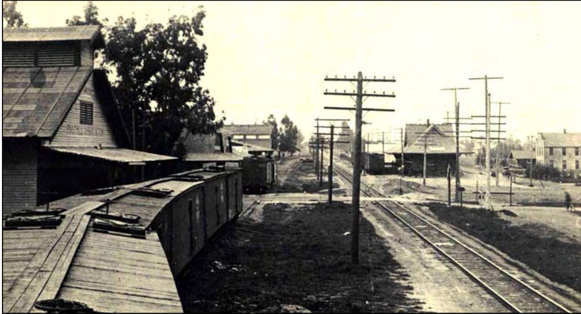
Fig. 7: View northwest, Intersection of 8th and Archibald Avenue along Santa Fe Railway c. 1900 (Clucas, Donald L. Light Over the Mountain: A History of the Rancho Cucamonga Area. Upland: California Family House, 1979, 77).
