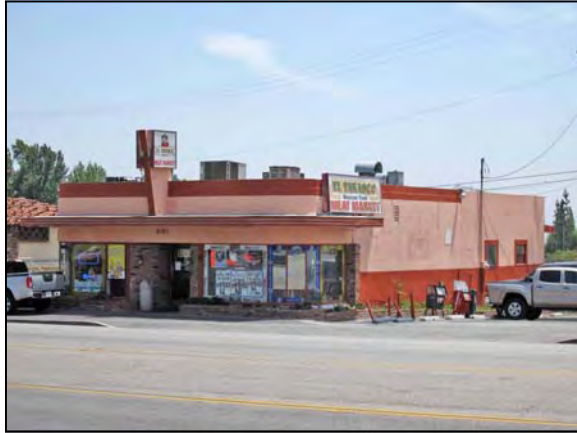
Fig 1: Foothill Liquor, 8161 Foothill Boulevard (c. 1945) (Chattel Architecture 2009)
