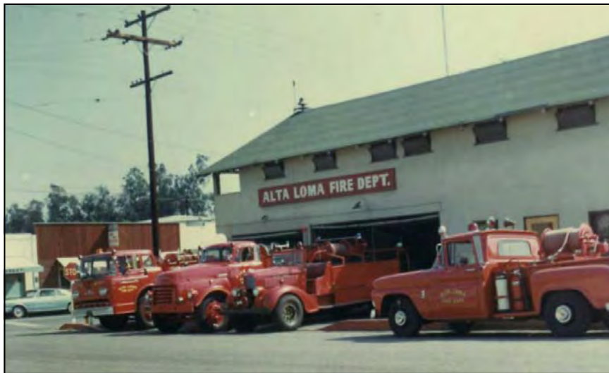
Fig. 4: View southeast showing north elevation of Alta Loma Fire Hall (constructed c. 1931) facing Amethyst, note commercial store (now demolished) between historic Roth's Store and Post Office (Ernie's Place) and Billings Store on Amethyst Avenue behind Fire Hall (photo taken c. 1960; source unknown)
