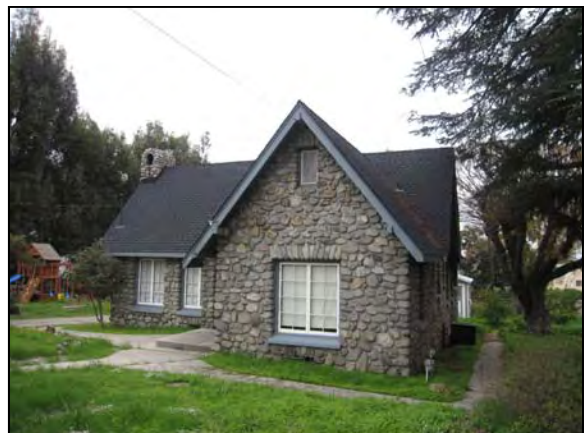
Fig 9: Alta Loma, typical example of stone construction in Alta Loma, located on south side of Hillside Road (Chattel Architecture 2009)
