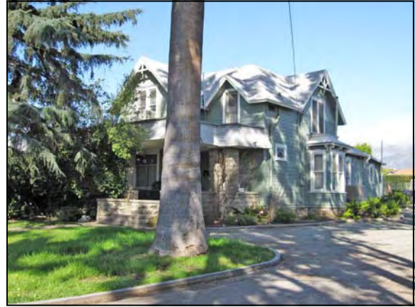
Fig. 11: View northwest of Cucamonga Rooming House, 9680 San Bernardino Road (c. 1900) (Chattel Architecture, 2009).
