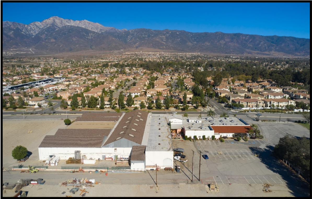
Overhead View of Winery Building Looking North
