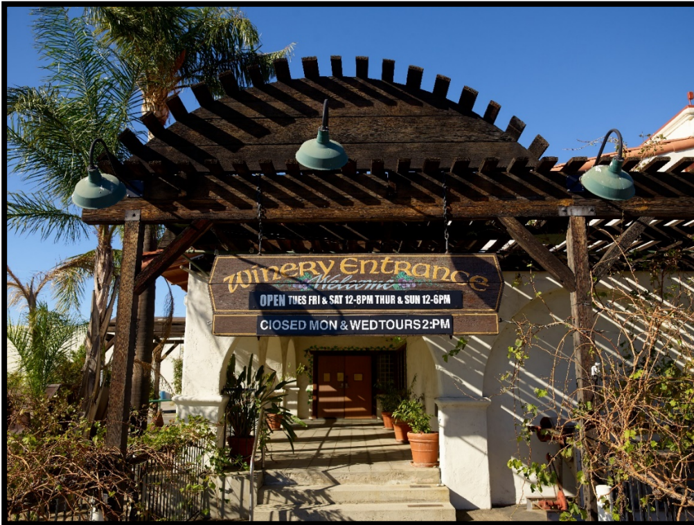
Front Elevation of Winery Building, View from Base Line Road
