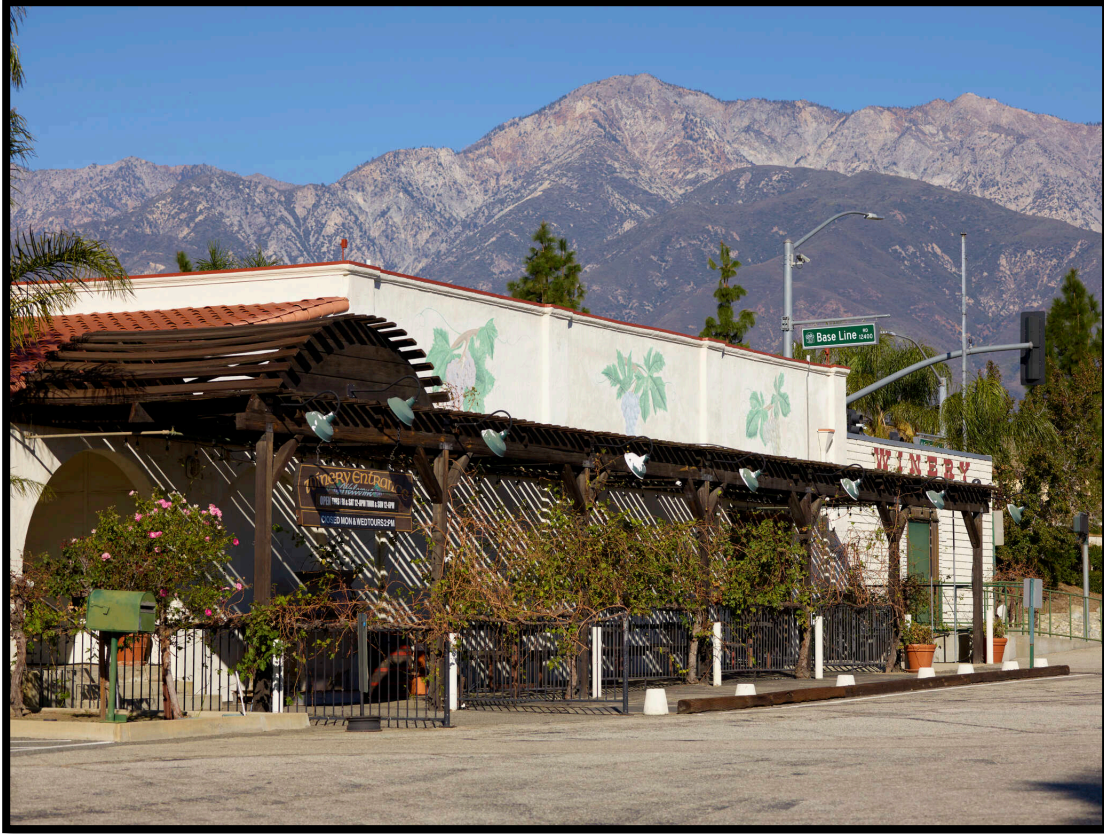
East Elevation of Winery Building
