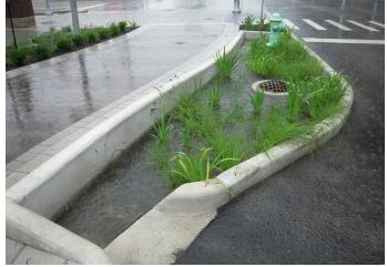
Storm infiltration system in bulbed corner
