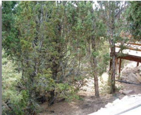
Flammable vegetation leading to deck
