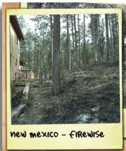
Fire burned very close to this home in New Mexico without igniting the wood walls.
