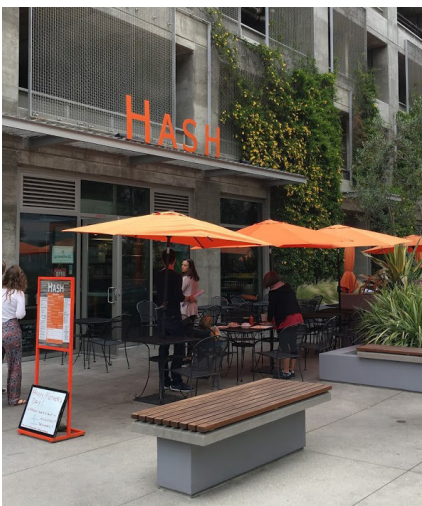
Cafe in parking structure "liner space"
