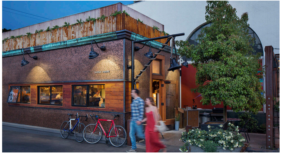
Adaptive re-use of a former industrial building into an eatery
