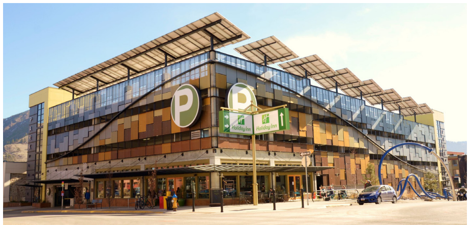
Parking structure artfully screened, and shaded with solar panels
