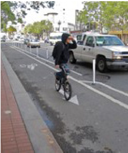
Protected bike lane
