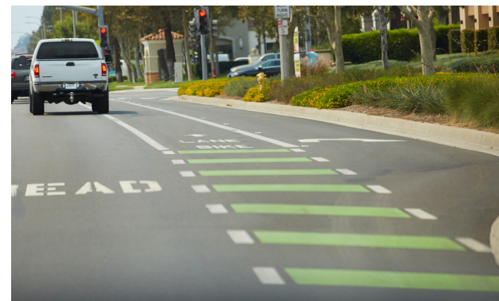
Example of bike lane striping near intersection to reduce conflicts.
