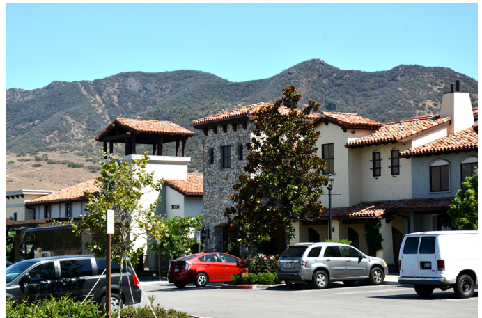
Varied massing and architecture creates sense of place
