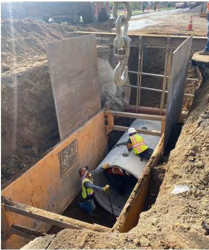
Upper Cucamonga storm drain
