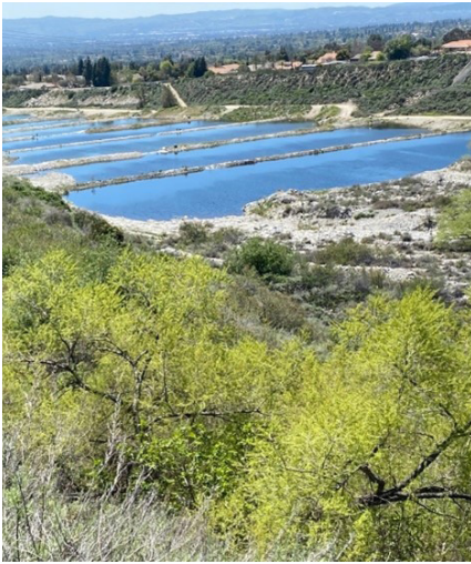
Open water catch basin
