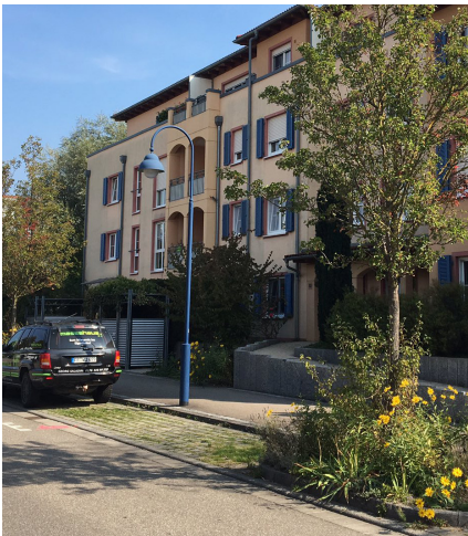
Parking lane planter and permeable paving
