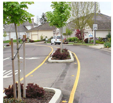
Lemon Avenue, which has house fronts, is a wide roadway, allowing cars to speed freely. Introducing medianettes is one way to encourage cars to drive more slowly and carefully through this neighborhood, in addition to improving the environmental quality.
