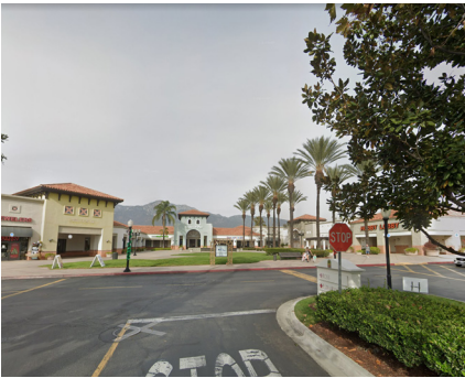
Many of our commercial frontages, while attractive, are disconnected from the public realm network by large parking lots.
