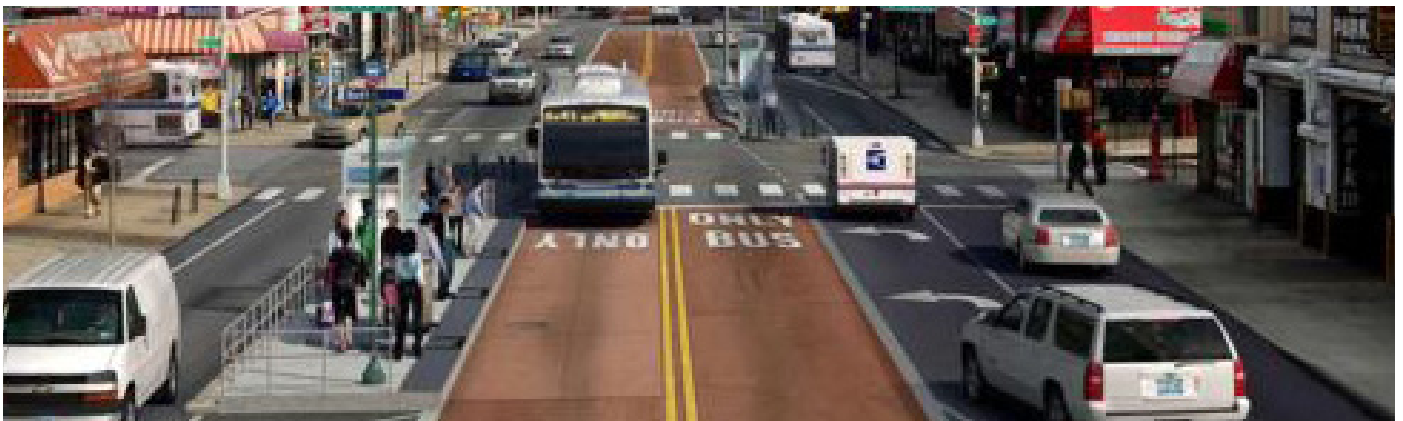
Striped median busway with raised platform bus stop
