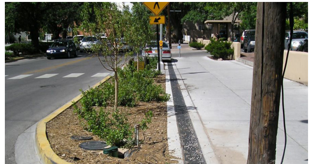
A mid-block bulb-out protecting a pedestrian crossing.
