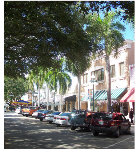
Frontage lane provides a high-quality and safe public frontage off of a busy corridor.
