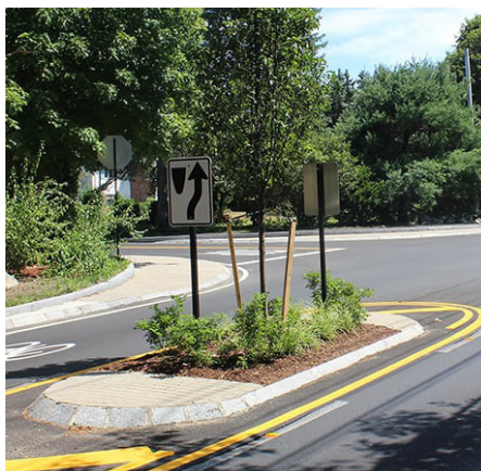
Lemon Avenue, which has house fronts, is a wide roadway, allowing cars to speed freely. Introducing medianettes is one way to encourage cars to drive more slowly and carefully through this neighborhood, in addition to improving the environmental quality.
