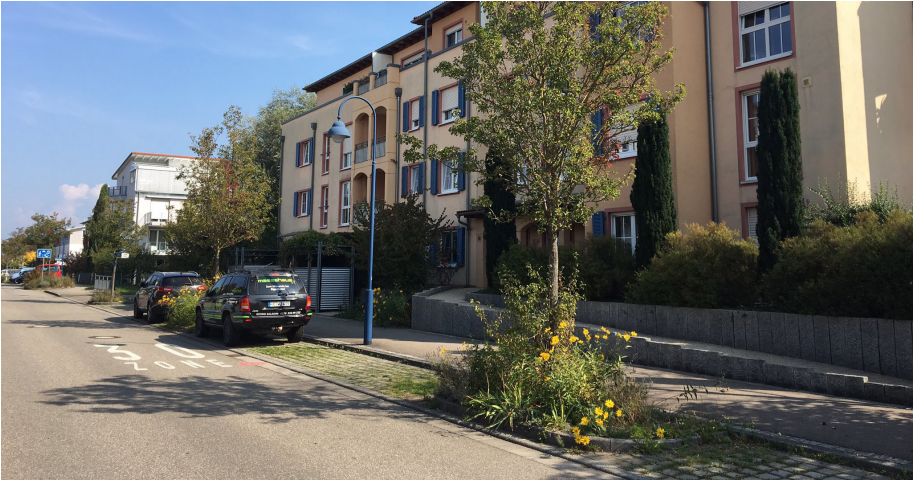
Parking lane planter and permeable paving in parking lane
