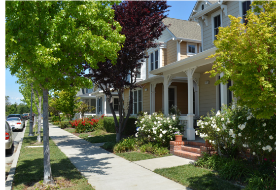
Example of semi-private yards and porches within the Front Setback Zone on a neighborhood street.
