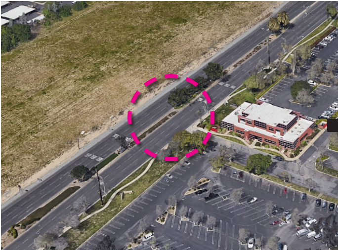
New signalized intersection needed
