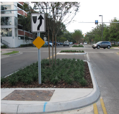
Lemon Avenue, which has house fronts, is a wide roadway, allowing cars to speed freely. Introducing medianettes is one way to encourage cars to drive more slowly and carefully through this neighborhood, in addition to improving the environmental quality.
