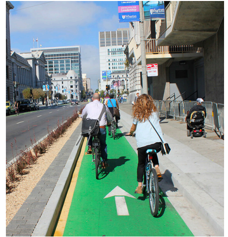
Protected bike lane
