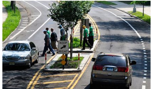
Mid-block crossing with a medianette pedestrian refuge.
