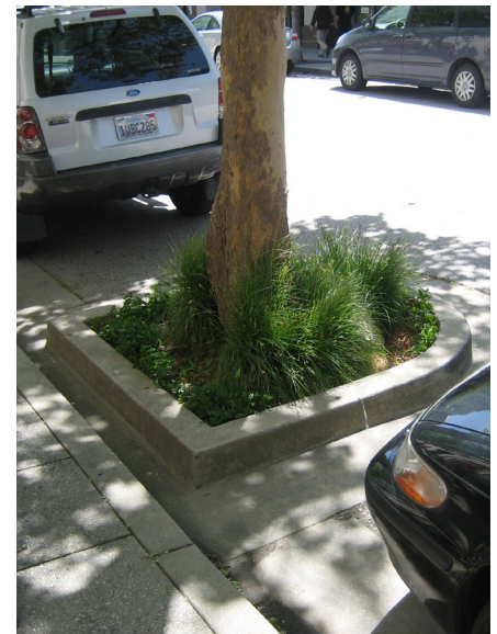
Tree planter in Curbside between on-street parking
