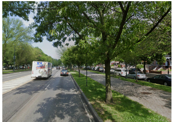
Wide median between frontage lane and travel lanes
