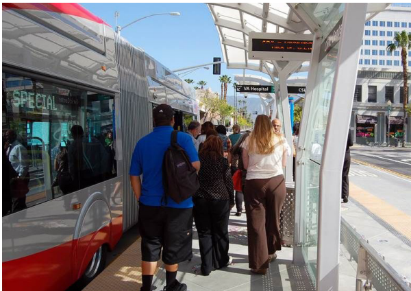
Barrier and shade structure at median boarding island
