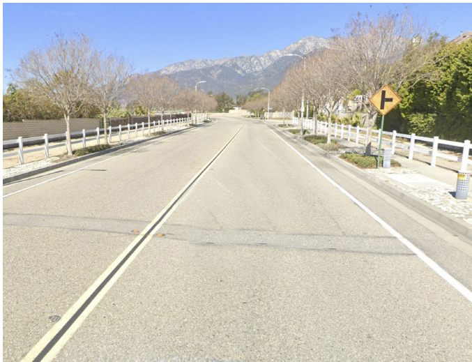
Existing bike lane on Highland Avenue is not well protected from vehicular traffic and could be improved with a buffer.
