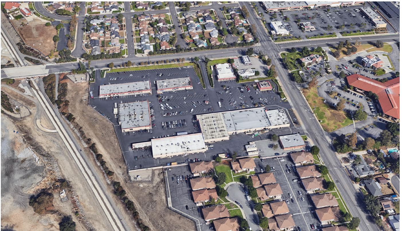
Case Study #2 Site seen from the southwest
