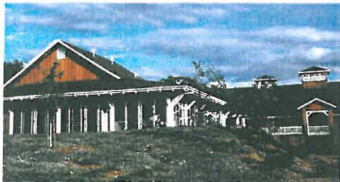
THE MUMM WINERY - NOTE USE OF ARCADES TO BRING BUILDING DOWN TO PEDESTRIAN SCALE.
