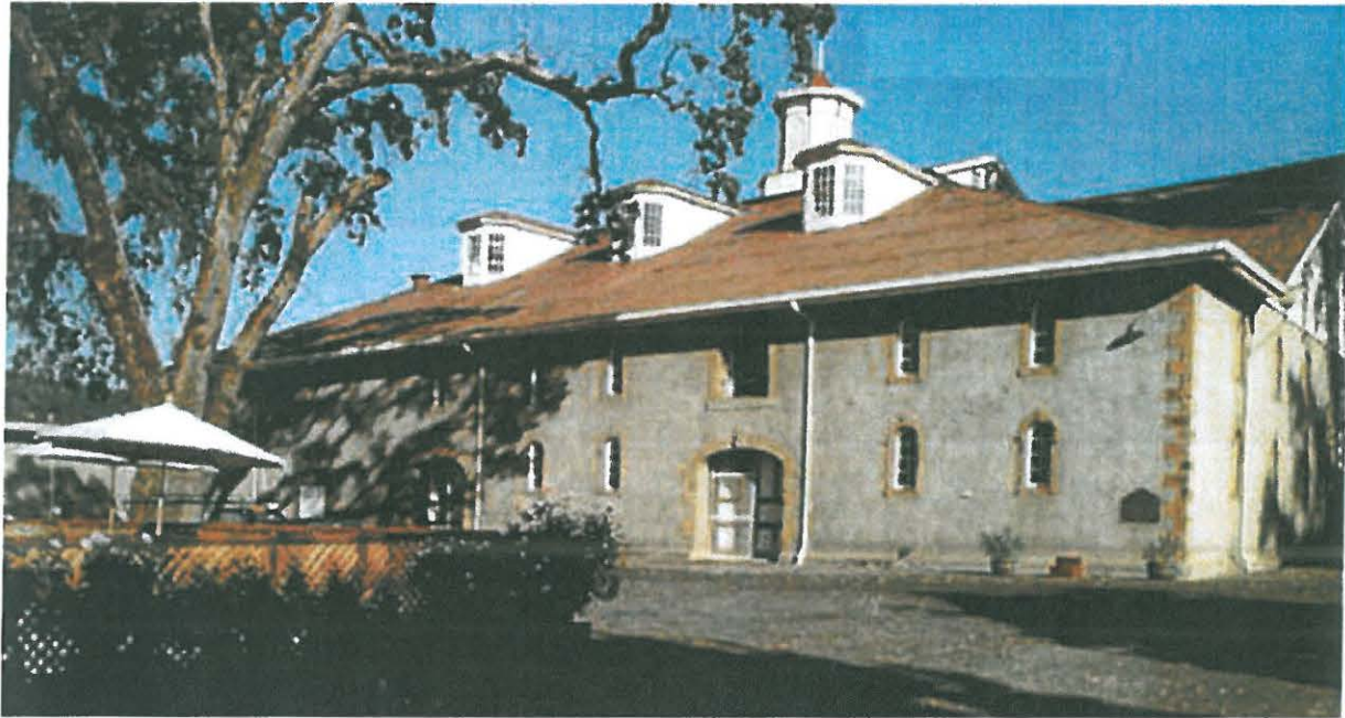
CHARLES KRUG WINERY - NOTE ROOF TREATMENT, WINDOW TREATMENT AND MATERIALS.
