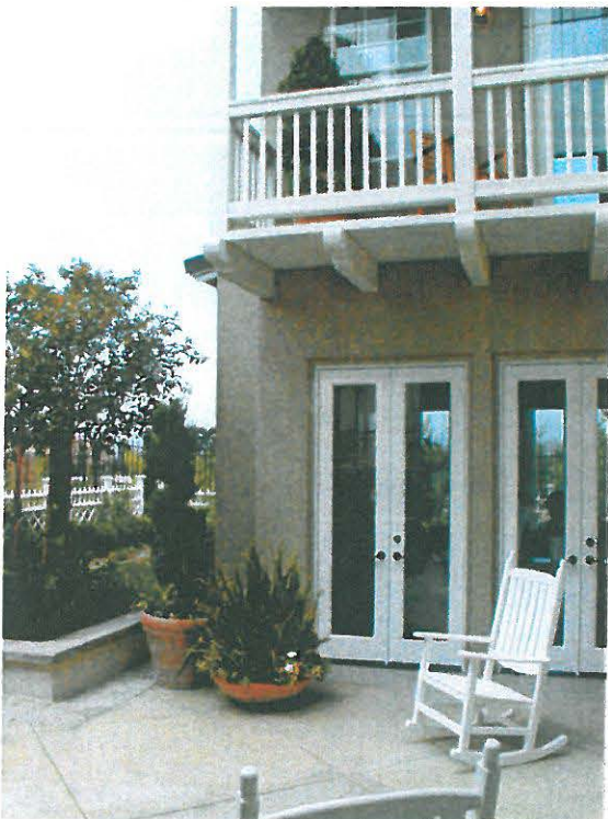
Balcony Provides Shelter over First Floor Doors
