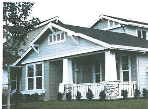
A Large Porch - Good Building Detailing
