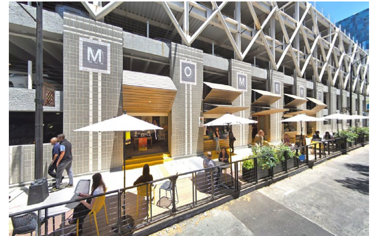
Large shared parking structure with micro-retail liner
