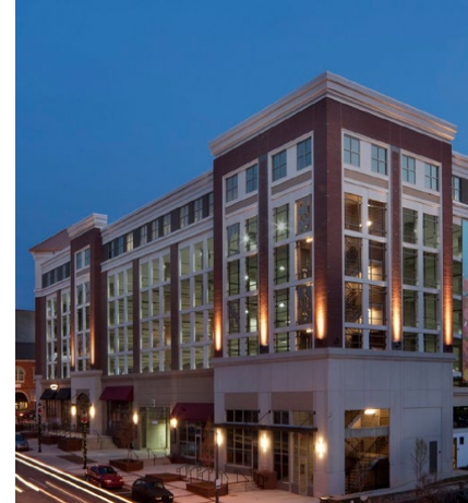
Large parking structure with ground floor retail liner
